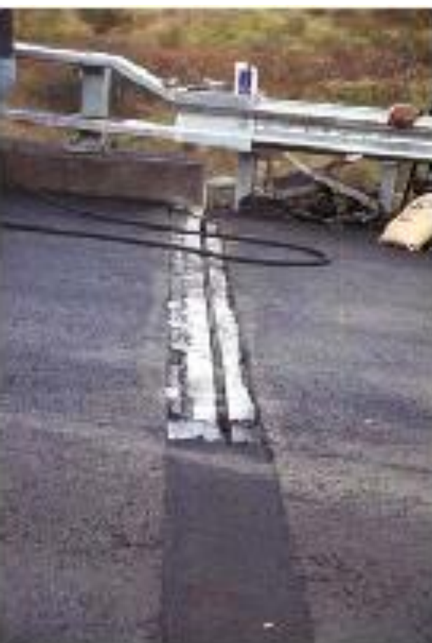
Figure 5.4.12 Asphaltic Expansion Joint
