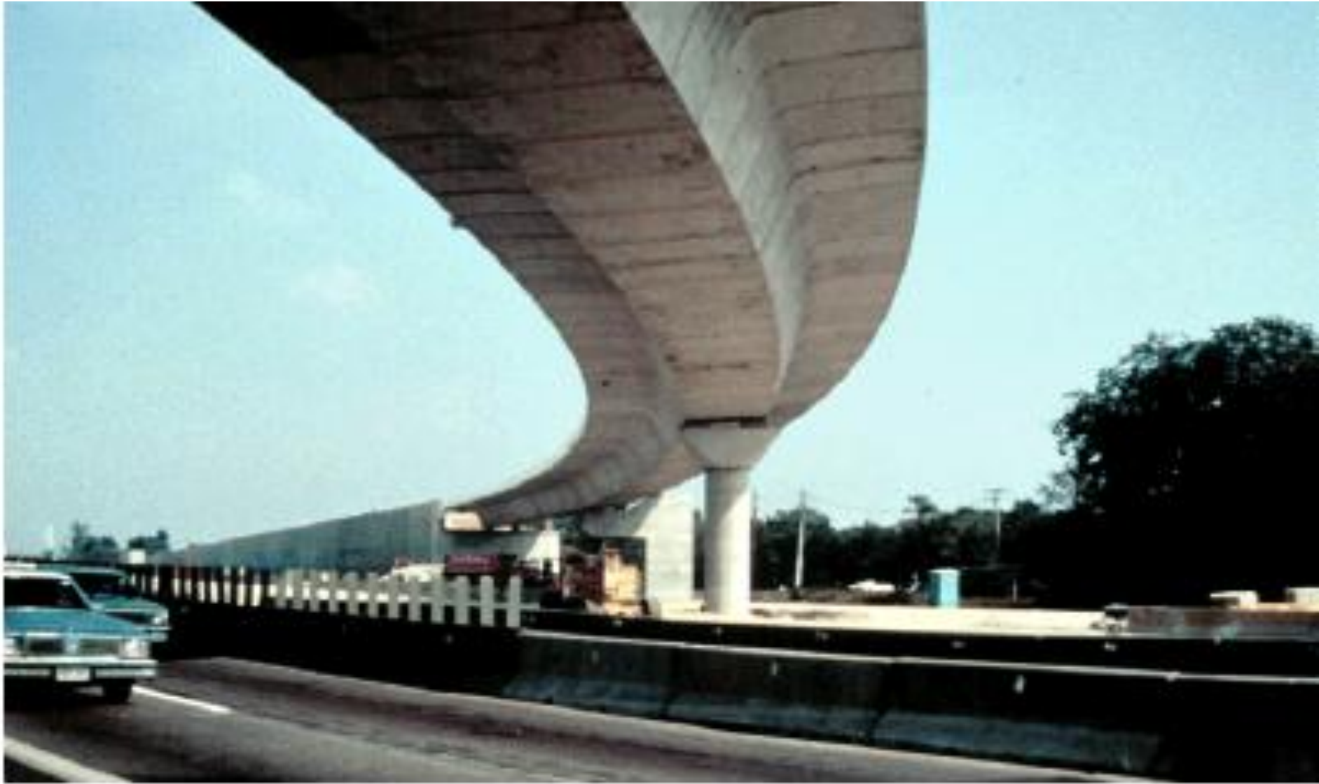
Figure 7.11.12 Segmental Concrete Bridge
