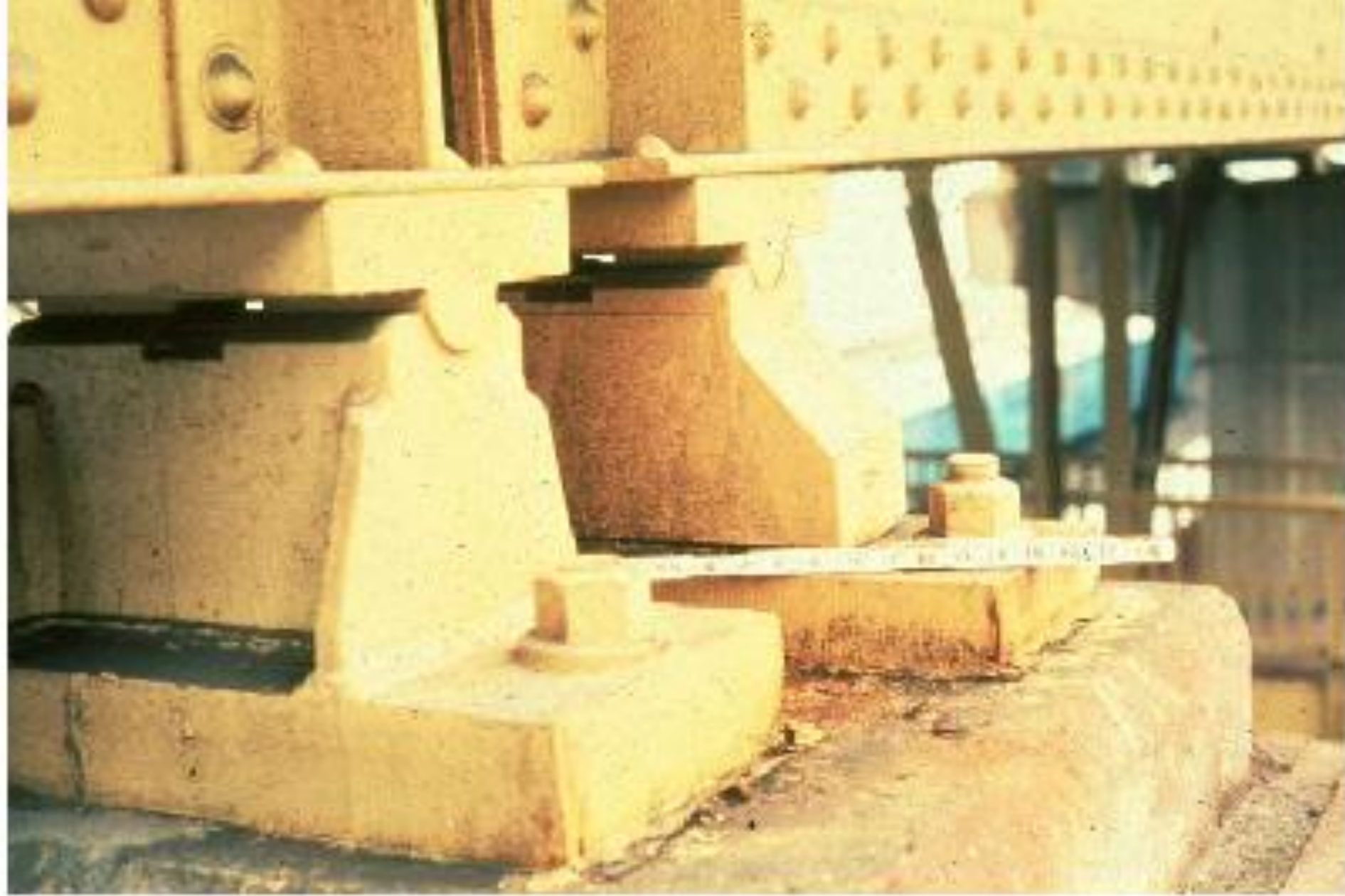
Figure 9.1.2 Fixed and Expansion Bearings
