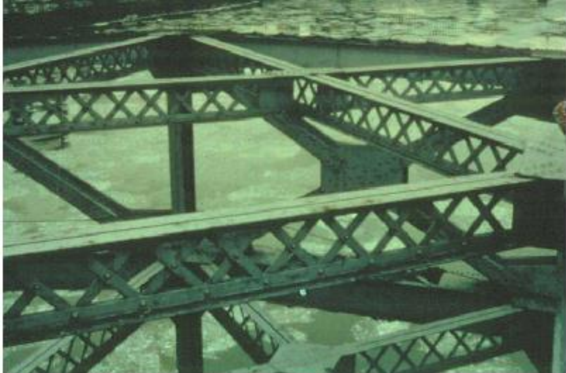
Figure P.2.12 Bracing Members Made from Angles, Bars, and Plates
