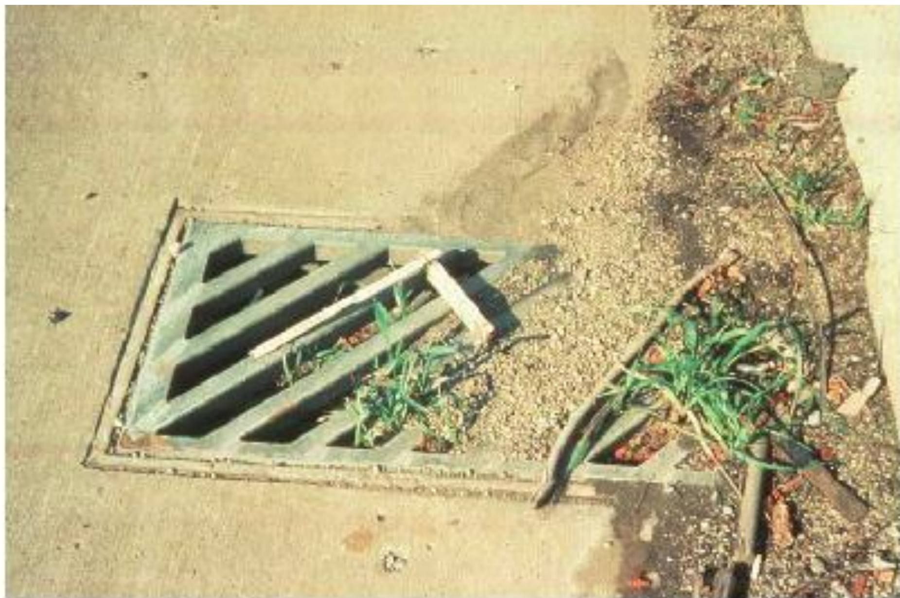
Figure 5.4.13 Bridge Deck Inlet
