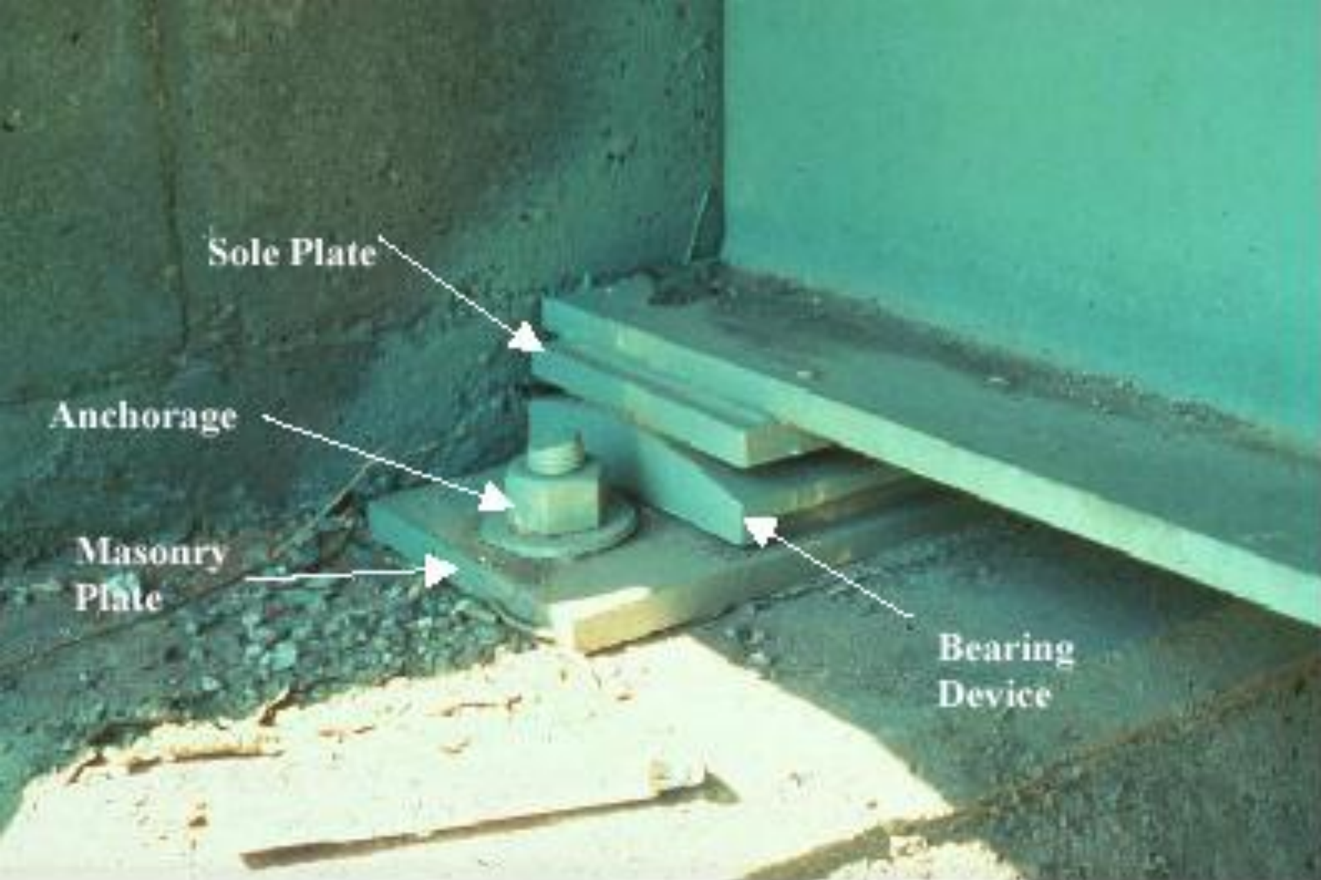
Figure P.2.64 Typical Bearing Showing Four Basic Elements
