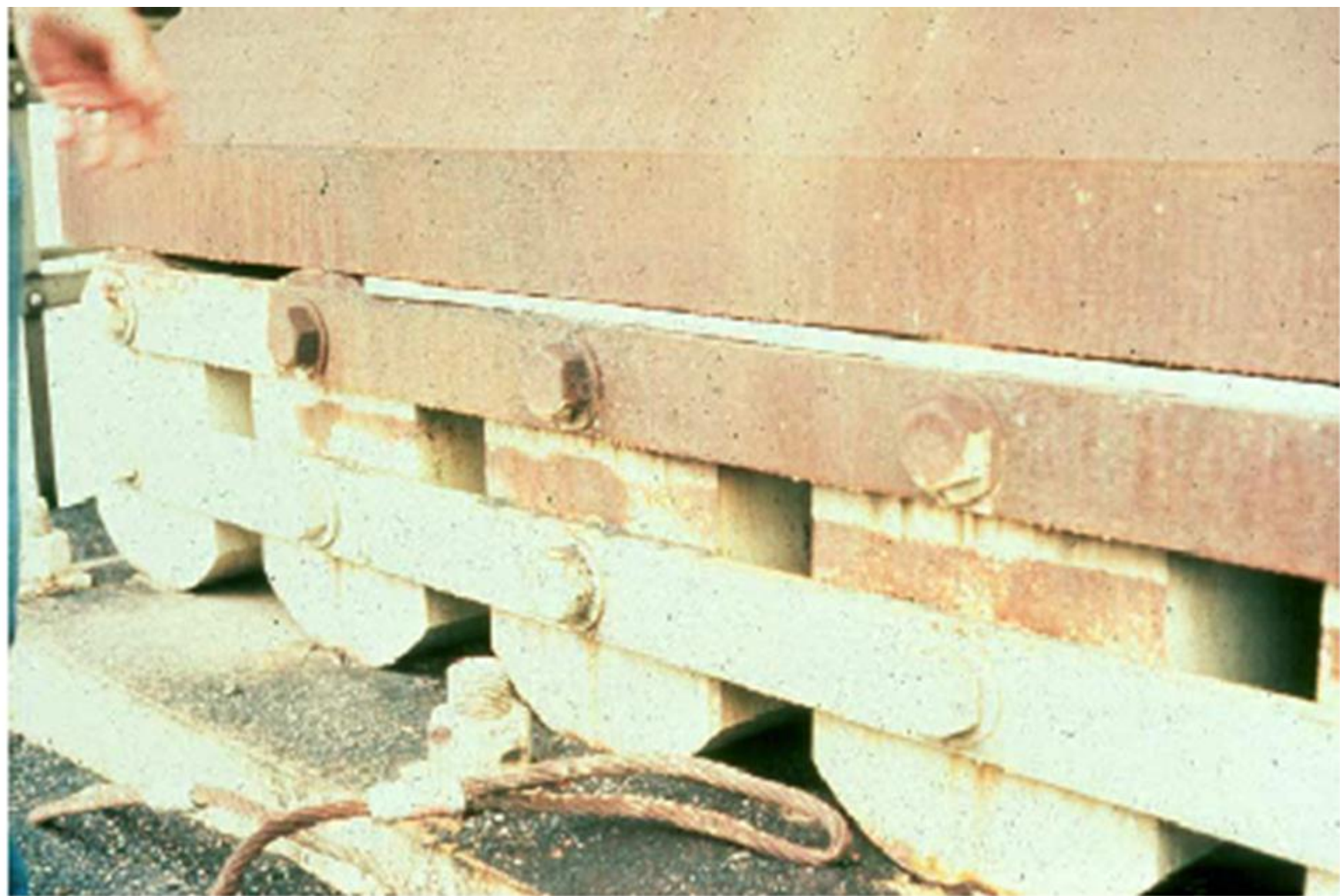
Figure 9.1.11 Segmental Rocker Nest Bearing
