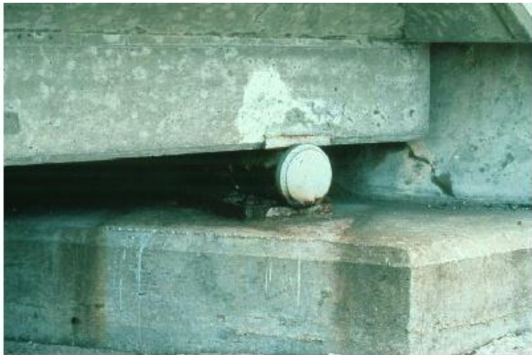
Figure 9.1.7 Single Roller Bearing
