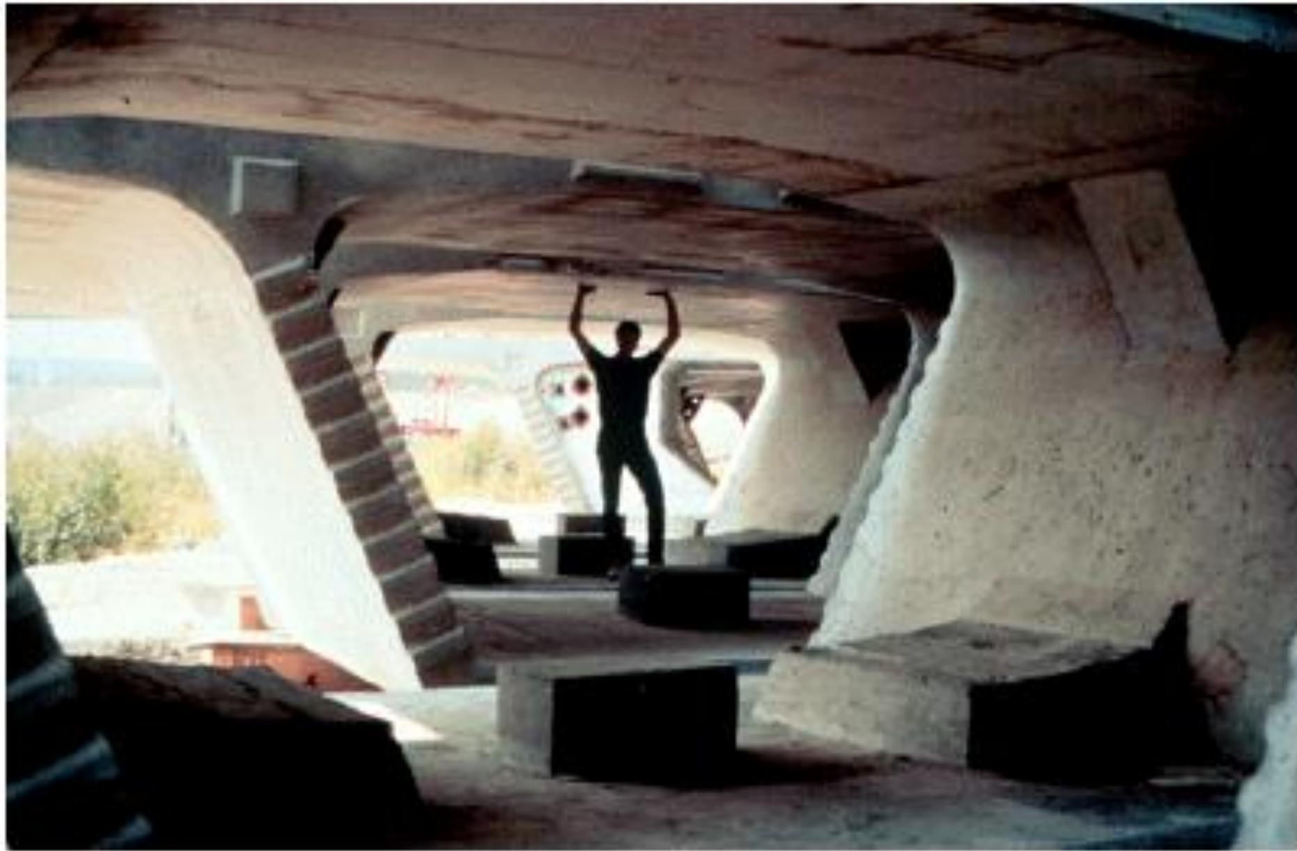
Figure 7.11.15 Box Girder Segment
