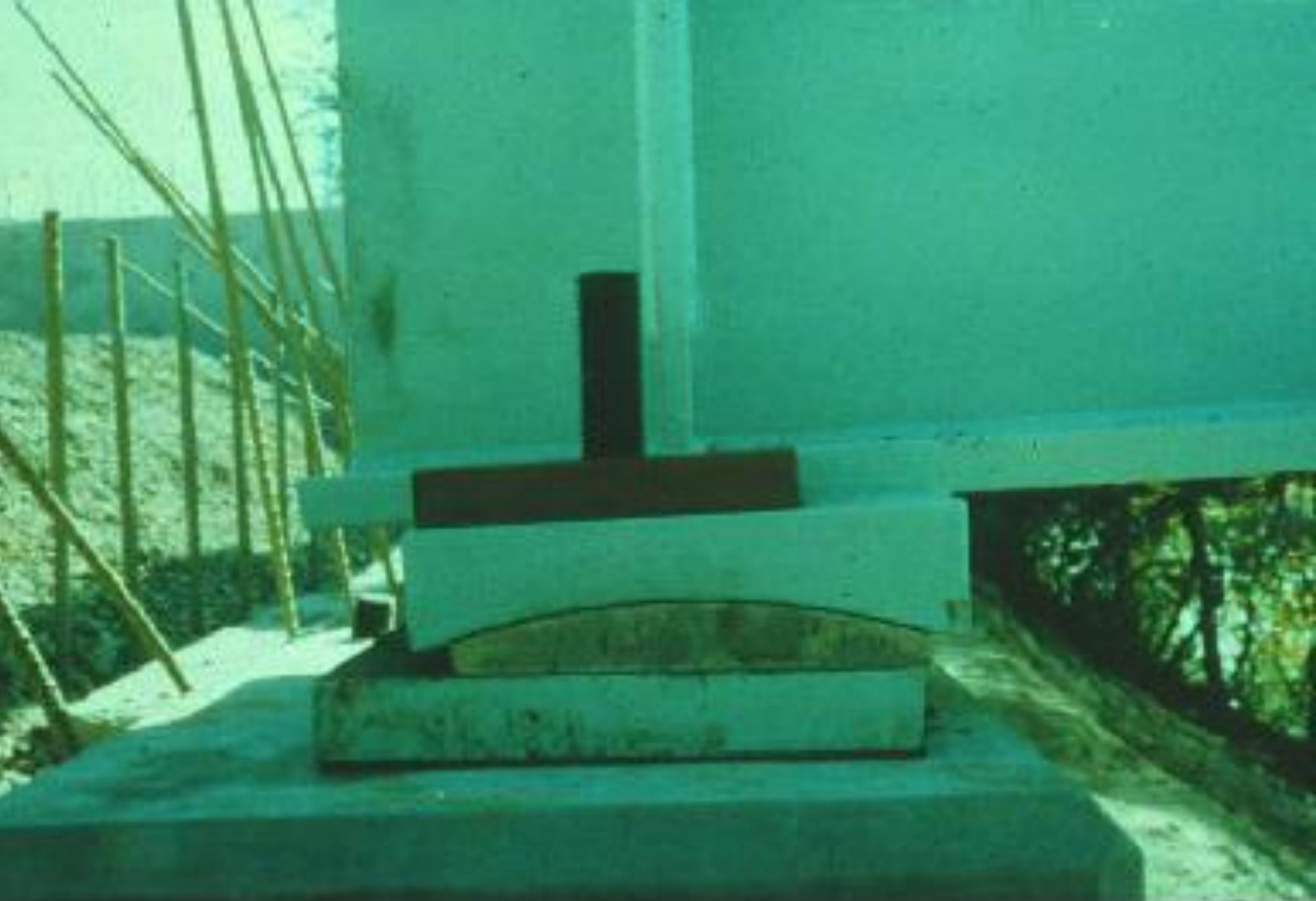
Figure 9.1.5 Bronze Sliding Plate Bearing
