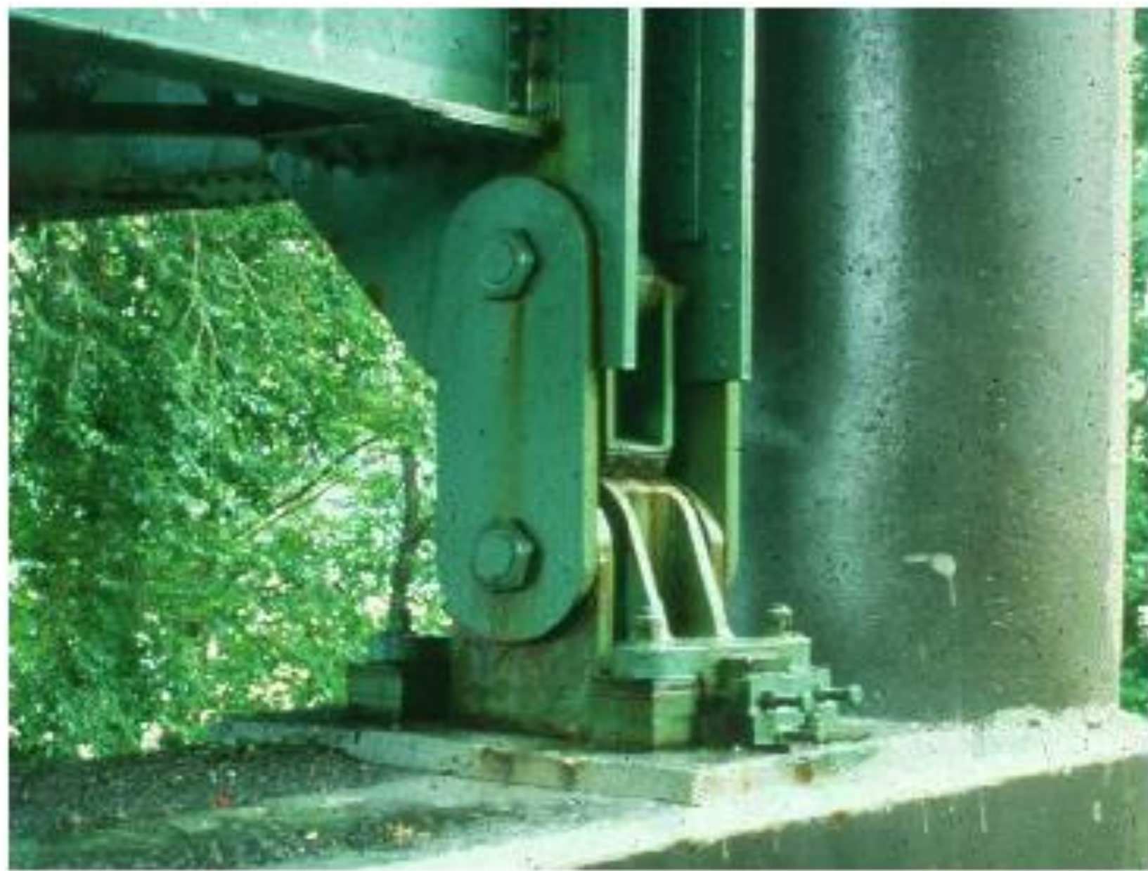
Figure 9.1.13 Pin and Link Bearing
