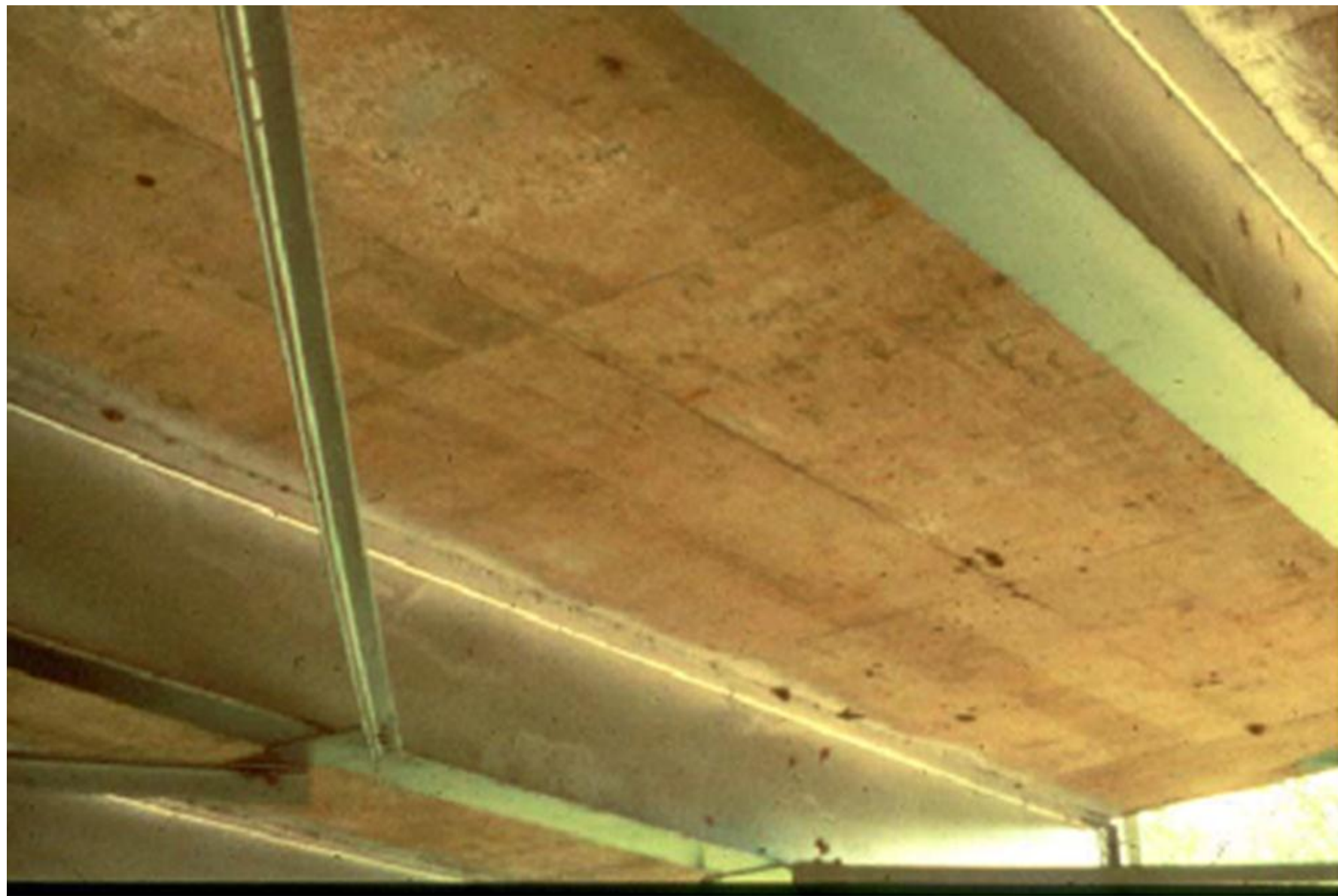
Figure P.2.30 Concrete Deck
